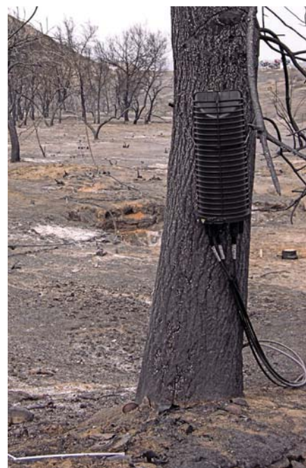
Some fiber survived. Here is a temporary fix. Courtesy of Jim Hayes
