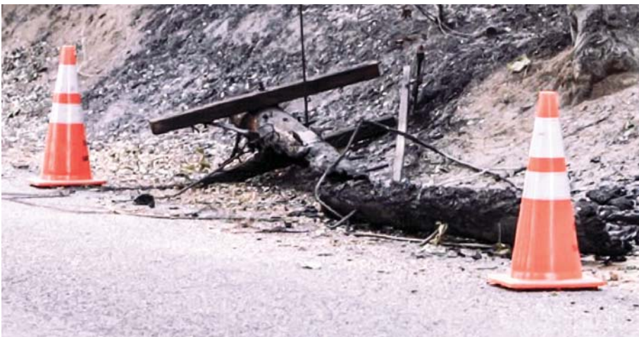
A wooden utility pole after a wildfire. Courtesy of Jim Hayes
